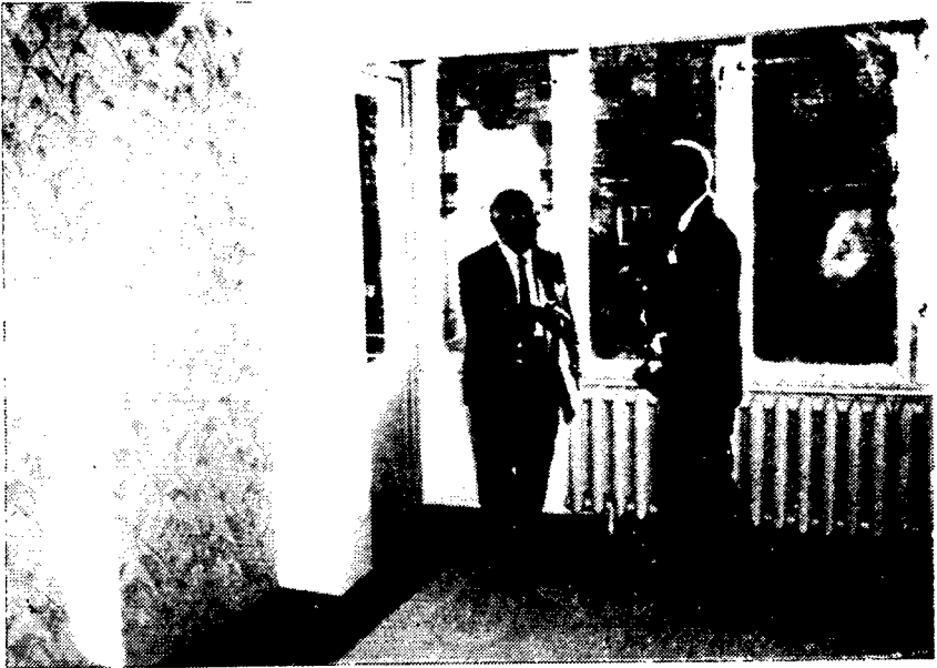
7. Details of interior finishing in new Soviet apartment. Papered and painted walls, hardwood parquet floor (partly covered by felt mat), hot water radiator, prefab glassed-in balcony.
